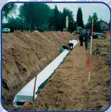
Pervious Swales using E.S.S. Modular Geo-Cell System for large and efficient movement of water.
