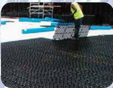
Installation of E.S.S. GeoCell 52 .
