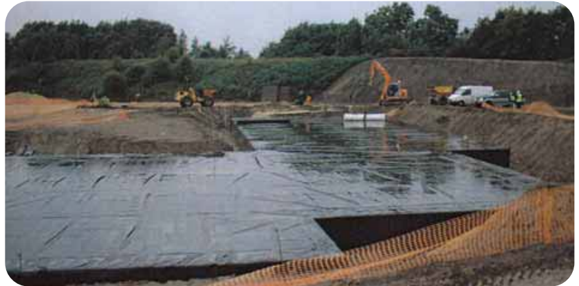
Attenuation Tank under Park and Ride Scheme showing versatility of modular system.
